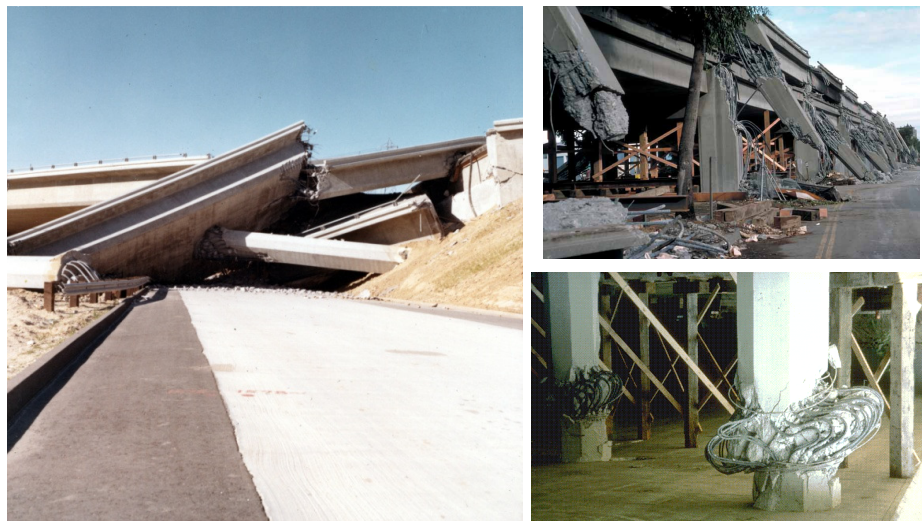
Figure 1-2: Earthquake damage: San Fernando (left); Loma Prieta (top right); Northridge (bottom right) [photos accessed through USGS website (2009)]
