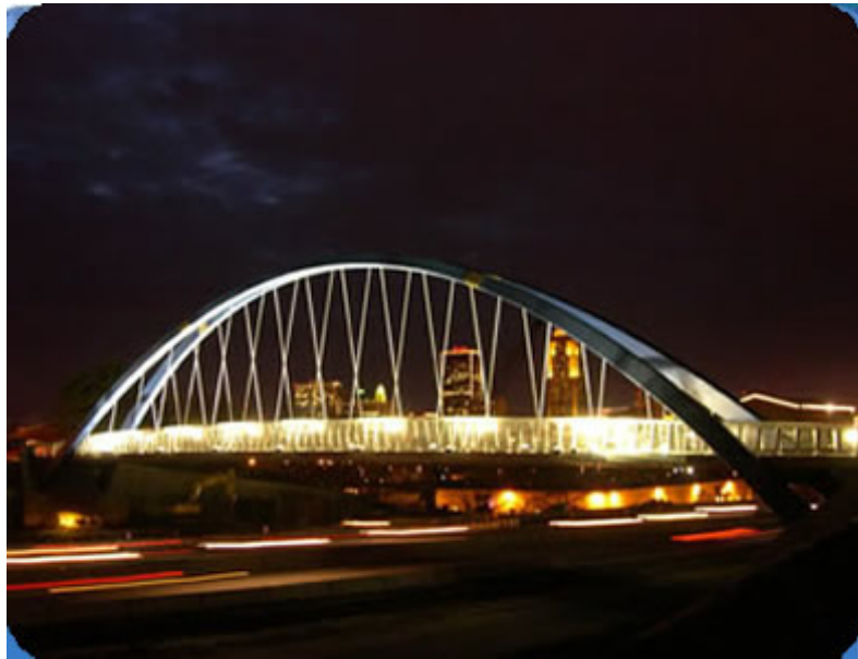
Figure 1-1: Arched pedestrian bridge over I-235 in Des Moines, Iowa (Iowa DOT, 2009)
